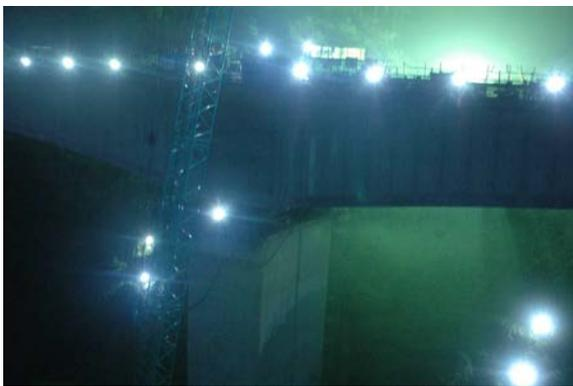
Fig.5: LED lights attached to a highway bridge under construction
