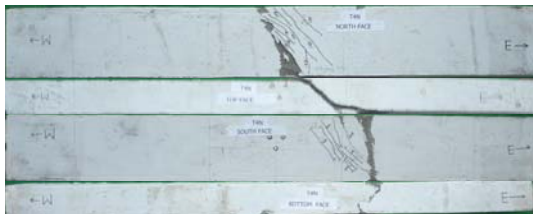
Fig. 5 Crack Pattern of T4N
