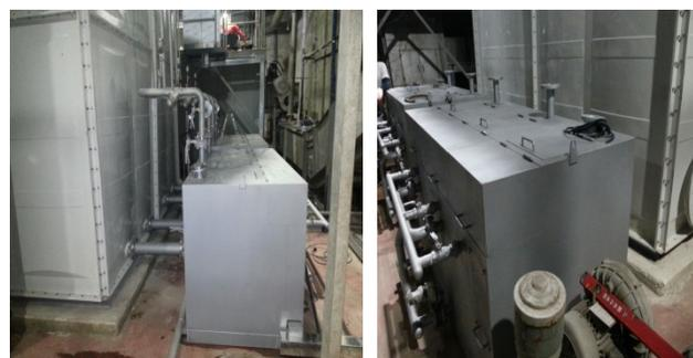
Fig. 3 Microorganism circulatory flask of actual biofilter
