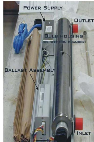
Fig. 3 Schematic of UV unit with cover removed [11]
