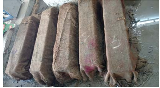
Fig 9. Curing using gunny bags
