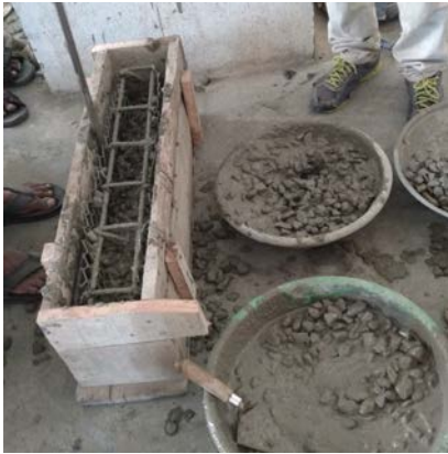
Fig 6.Placing of Concrete
