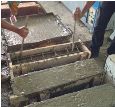
Fig 7. Compaction of Concrete
