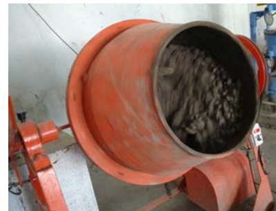
Fig 5. Mixing of Concrete
