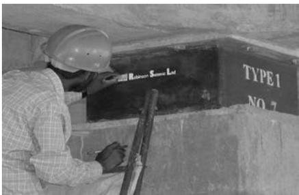
Fig. 2 Lead Rubber Bearing designed by Bill Robinson
