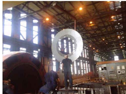
Figure 4. Monolithic end pack of the stator magnetic core in the process of mounting for turbo-generator n.1 in TPP Bitola
