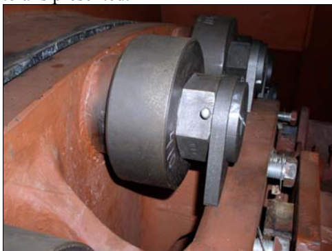
Figure 6. Pressure accumulator mounted on turbogenerator n.1 in TPP Bitola
